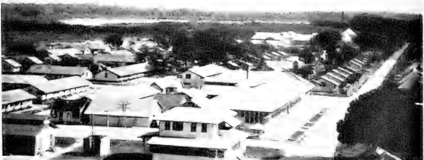
2. Moengo, Surinam. Practically every square foot of surface of these buildings was sprayed with a 2.5-percent wettable DDT powder.
